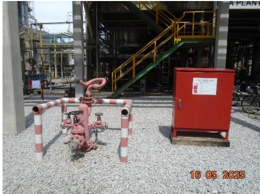
Water Hydrant/Fix Monitor
